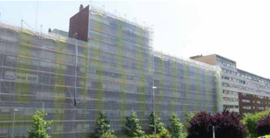
► Building in the Canyelles neighbourhood - BARCELONA
